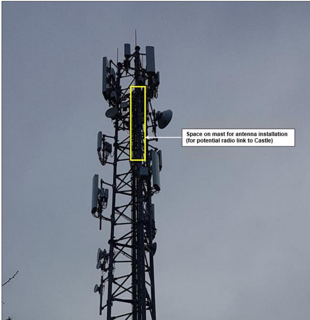
**Figure 15. Available space on Creevagh Telecoms Mast for potential radio link to Castle.**
