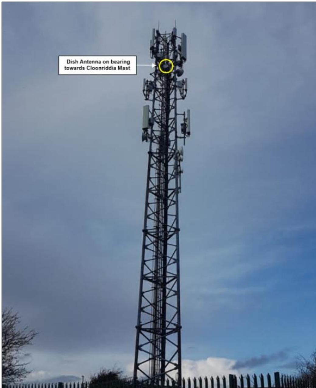
**Figure 14. Existing radio link from Creevagh to Cloonriddia.**
